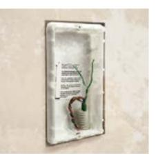
Use of an existing pair of wires to connect the new 2 Wires entrance panel
